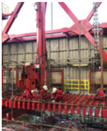
Aker-MH bridge crane & fingerboard inspection & repairing
