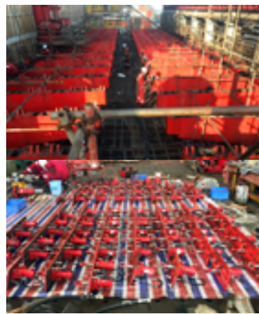
Aker-MH riser fingerboard inspection & repairing
